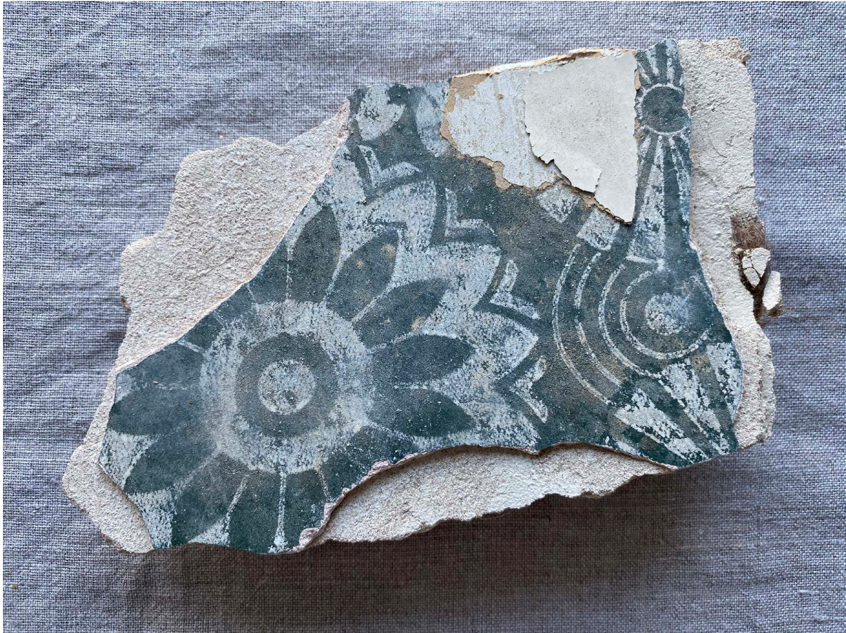
Painted wall decoration from front sitting room – c. 1800s [?] – cream paint stencilled using a stipple brush onto dark green
