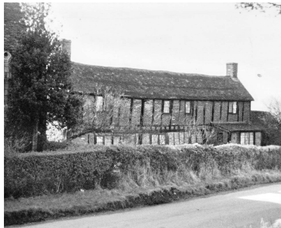
A picture of Pilgrim's Cottage taken in the late 1970s showing how the first floor is out of alignment with the ground floor
